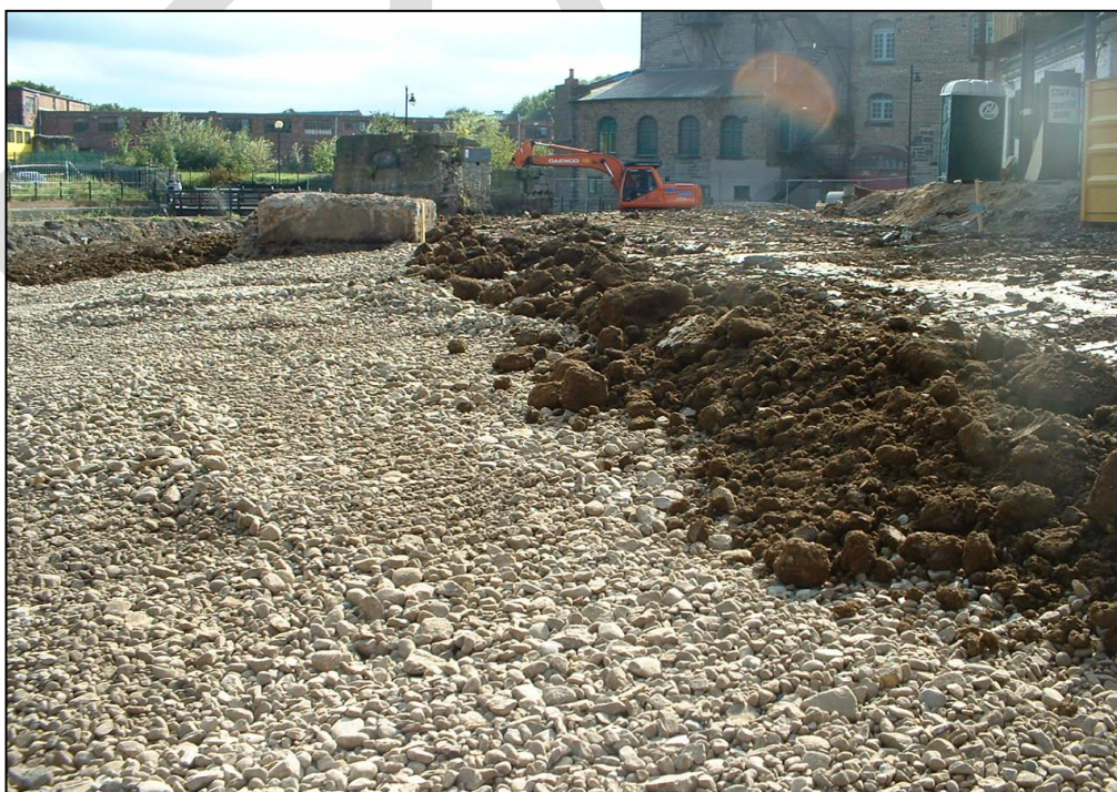
Former Byker City Farm. Placement of capillary break layer and clay cap.
