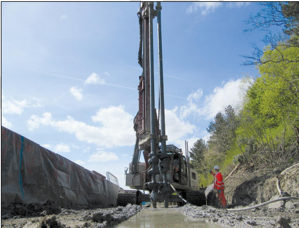
Installation of the soil mix barrier wall at St. Anthony's Tar Works
