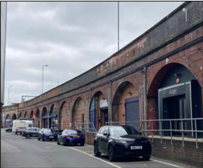
The viaduct arches on Forth Goods Yard.
