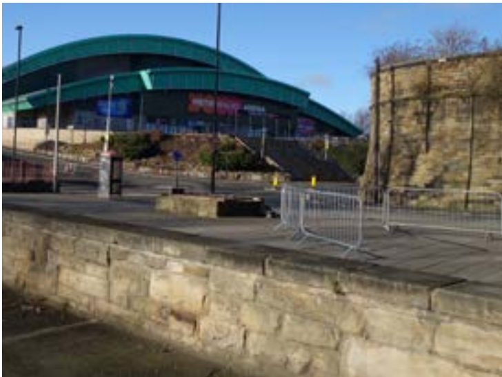
Sandstone Walls and changes of level that converge at the end of Pottery Lane after passing under Redheugh Bridge.
