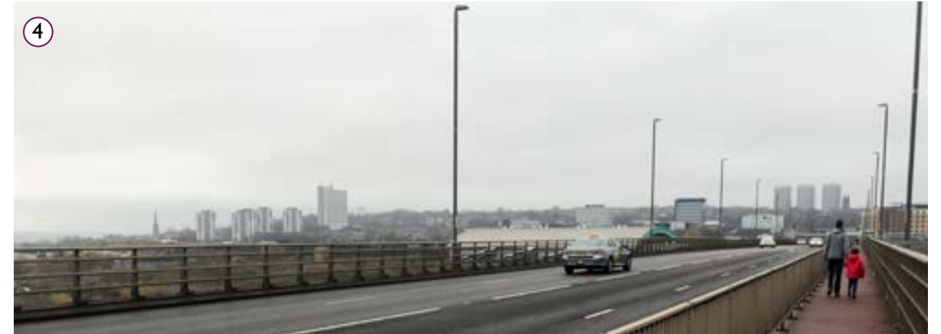
Looking across the Redheugh Bridge from the pedestrian walkway.
